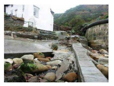
**Photograph 3.32** Runswick Bay 07-07A-02 Patch repairs with ad-hoc extension of wall and access to beach
