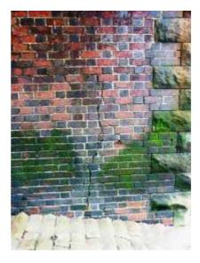
**Photograph 3.92** Filey Bay 67-28B-04. Vertical crack approx. 2m high
