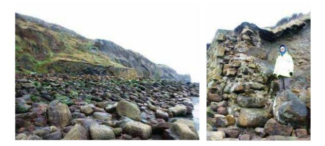
**Photograph 3.43** Gouldsborough 12-08B-01. Failed seawall with rock armour **Photograph 3.44** Gouldsborough 12-08B-01. Failed defence
