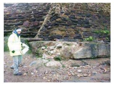
**Photograph 3.66** RHB 36-16A-01. Heavily abraded concrete apron
