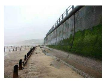
**Photograph 3.47** Sandsend 14-09B-05. Light scour at toe and dilapidated groynes
