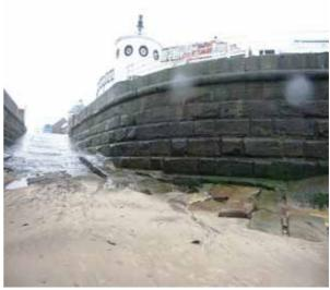
**Photograph 3.62** Whitby West Pier 26-11B-02. Uneven surface at access to walkway
