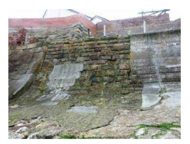
**Photograph 3.86** Cayton Bay 59-24B-01. Patch repairs and interface between different wall elements
