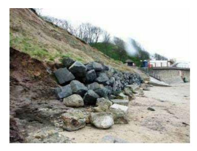
**Photograph 3.95** Filey Bay 67-28B-13. On-going coastal **erosion** and outflanking of defences
