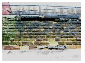
**Photograph 3.57** Whitby West Cliff 20-11A-02. Masonry blocks are missing just below the promenade
