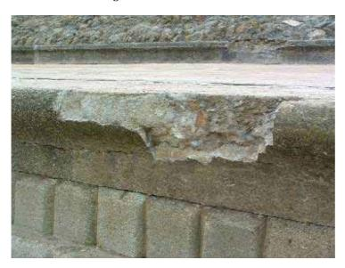
**Photograph 3.70** SNB 42-20A-09. Damaged wave return wall
