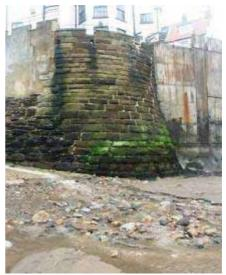
**Photograph 3.64** Robin Hood's Bay (RHB) 32-16A-02. Slipway with rocks partially covering access
