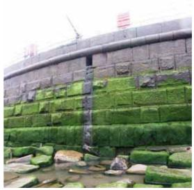
**Photograph 3.59** Whitby West Pier 22-11A-02 Abraded steps
