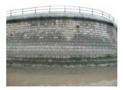
Photograph 3.94 Filey Bay 67-28B-07. Scouring at toe
