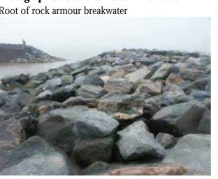
Photograph 3.22 Staithes Eastern Breakwater Rock armour revetment
