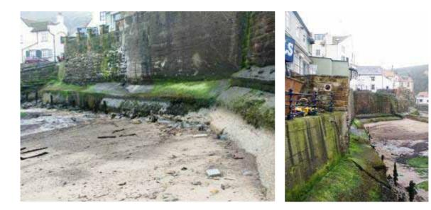
**Photograph 3.12** Staithes 02-04-01. Poor condition wall, missing blocks etc
