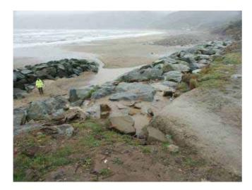
**Photograph 3.37** Runswick Bay 10-07B-01 Water running through rock armour onto beach
