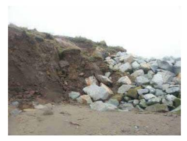
**Photograph 3.67** RHB 37-16C-03. Landslip partially covering defence asset
