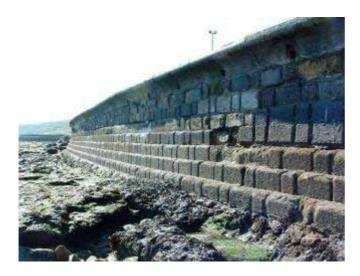
**Photograph 3.82** SSB 55-22B-01. Abraded masonry blocks
