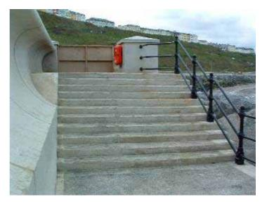
**Photograph 3.74** SNB defences south of asset 44-20B-05 show some sign of wear and have suffered some damage. They require some remedial repairs
