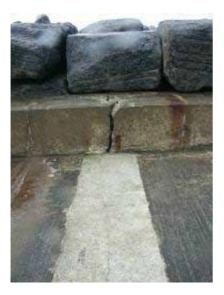
**Photograph 3.5** Staithes Northern Breakwater. Abraded and damaged concrete coping
