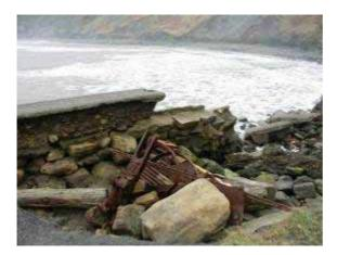
Only remnants indicate the former existences of a north breakwater and rock armour. Broken sections of this structure remain along the frontage. **Photograph 3.28** Port Mulgrave. Collapsed surface of south breakwater
