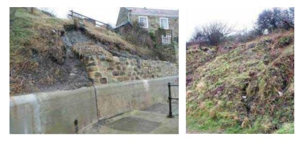
**Photograph 3.35** Runswick Bay 08-07A-03. Small slip onto the upper wall at promenade level.
