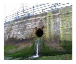
**Photograph 3.15** 03-04-01 Staithes. Damaged flap valves and cracked seawall.
