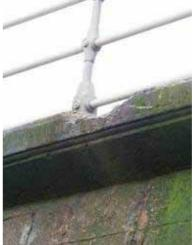
**Photograph 3.55** Whitby West Cliff 20-11A-01. Loose hand railing and scour
