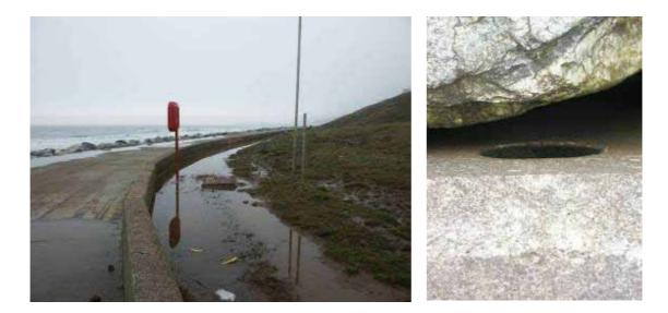
**Photograph 3.53** Whitby West Cliff 18-11A-02. Water standing behind the defence after a mild rain
