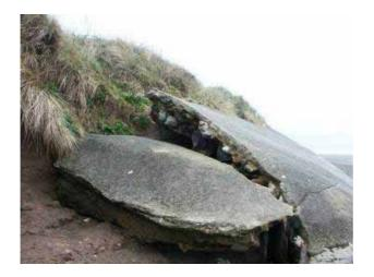
**Photograph 3.51** Sandsend Wyke 17-10-01 Undermined and partially failed Defence
