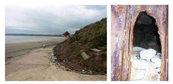
**Photograph 3.89** Filey Bay 64-28A-01. Landslide run-out lobe partially blocking the slipway
