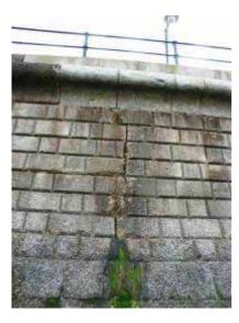
**Photograph 3.93** Filey Bay 67-28B-05 Vertical full height crack
