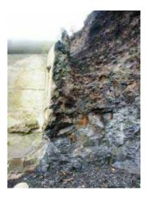
**Photograph 3.31** Runswick Bay 07-07A-01 Failed seawall section
