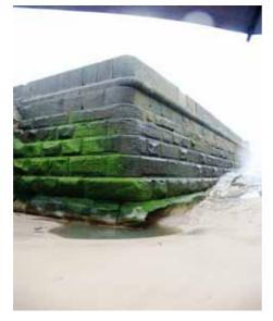
**Photograph 3.61** Whitby West Pier 26-11B-02. Scour at the base of harbour wall
