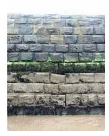
**Photograph 3.63** Whitby West Pier 27-11B-01. Blocks displaced due to movement.
