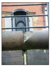
**Photograph 3.48** Sandsend 14-09B-01. Minor damage to wave return feature of wall
