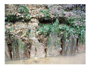
**Photograph 3.76** Scarborough West Pier (SWP) Timber toe piles and localised undermining
