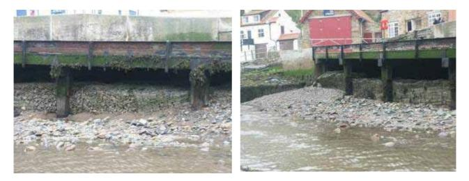
**Photograph 3.10** Staithes RNLI Slipway. Gabion Baskets beneath slipway **Photograph 3.11** Staithes RNLI Slipway. Gabion Baskets beneath slipway
