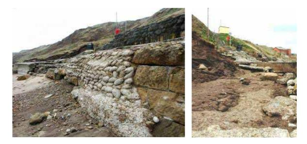
**Photograph 3.87** Cayton Bay 60-24B-01. Concrete bag-work and failed defence section. **Photograph 3.88** Cayton Bay 60-24B-01. Landslip and **erosion** below steps
