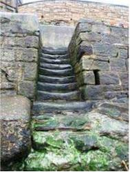
**Photograph 3.33** Runswick Bay 08-07A-01. Damaged apron in front of seawall
