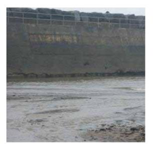
**Photograph 3.6** Staithes Northern Breakwater. Abraded vertical surfaces and toe scour
