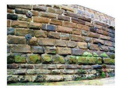
**Photograph 3.81** SSB 53-22B-05. Historical cracks and anchors
